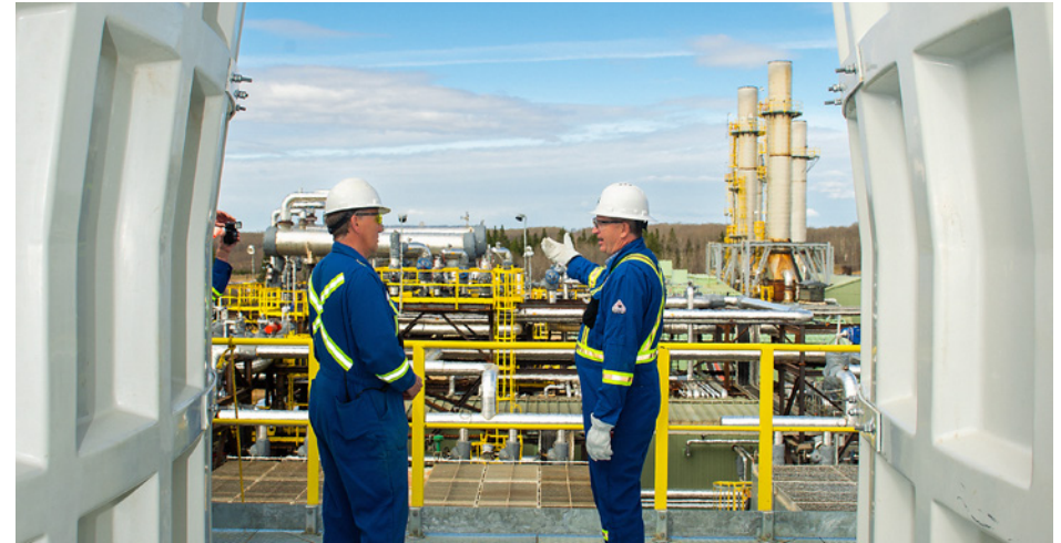
▲ Workers inspect the ORC's aerial cooling condensers during construction.
