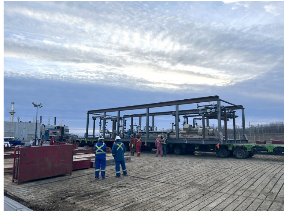
▲ Workers at our Lindbergh asset prepare to offload high-pressure injection/transfer pumps during construction activities for the OTSG upgrade. The upgrade will allow the OTSG to use produced water, reducing our freshwater needs.
