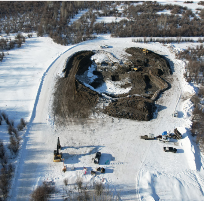
▲ Remediation efforts at the decommissioned battery and wellsite located within Hay Lake No. 209, Alta.
