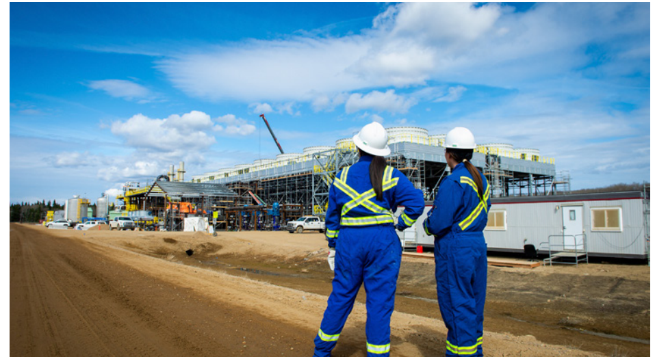
▲ Construction of the ORC nearing completion in spring 2025.
